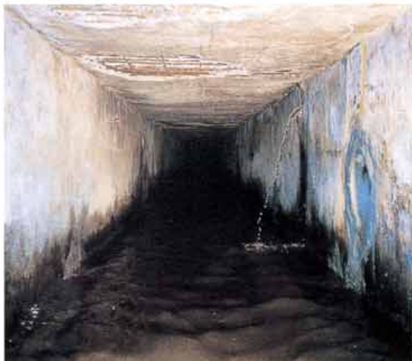
(Before renewal) (施工前)
