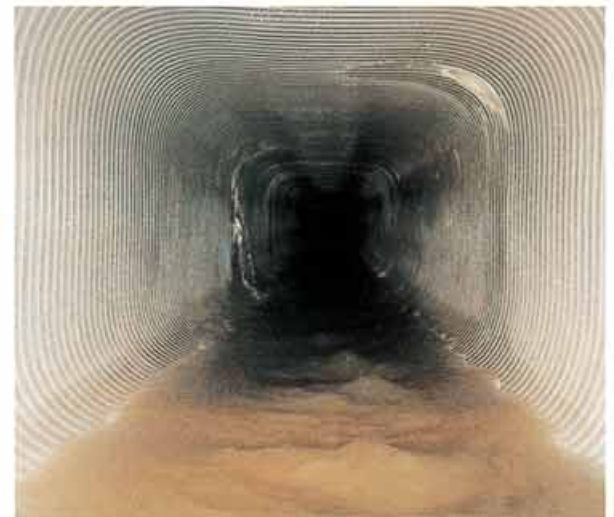
(After renewal) (施工後)
